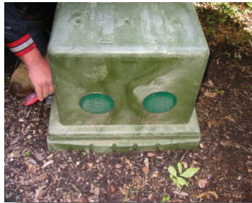
Developed to extend the life of leachfields, the commercially available SoilAir is now being tested for its ability to foster nitrogen removal as well.
